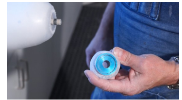
7. Remove tooling from anchor.
